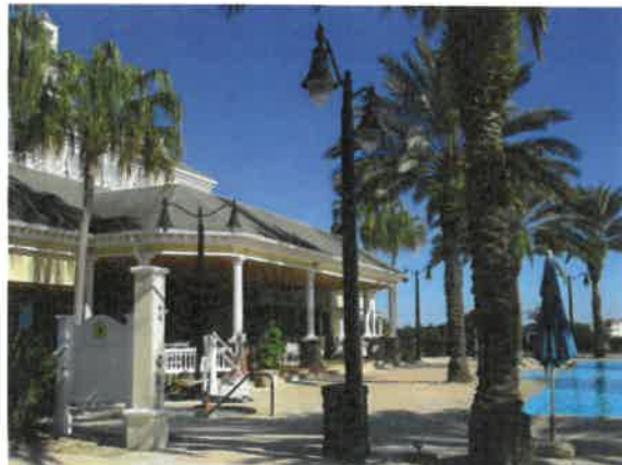
Light pole and fixtures at Seven Eagles
