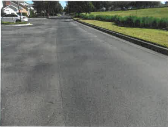
Asphalt pavement street at Heritage Crossing
