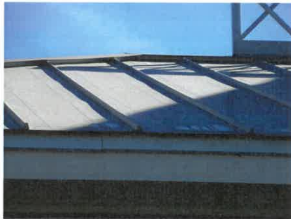
Standing seam metal roofing
