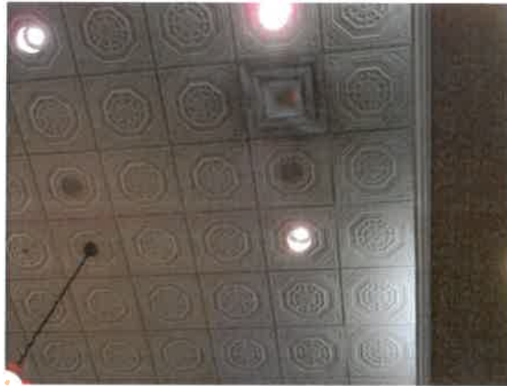
Acoustical ceiling tiles
