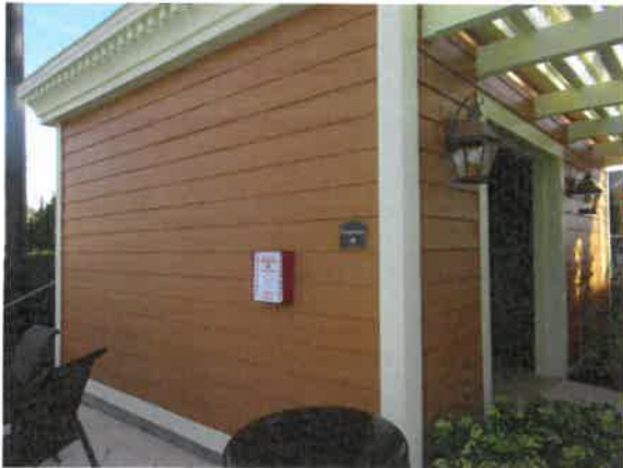
Fiber cement siding at Carriage Point pool house
