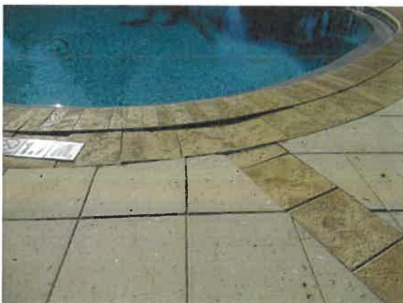
Isolated settlement at Homestead
