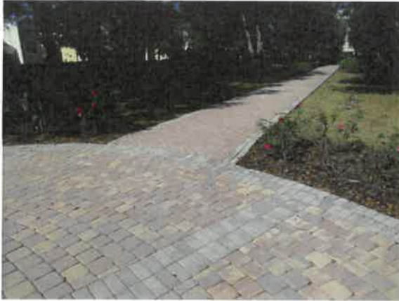
Masonry pavers at Seven Eagles park
