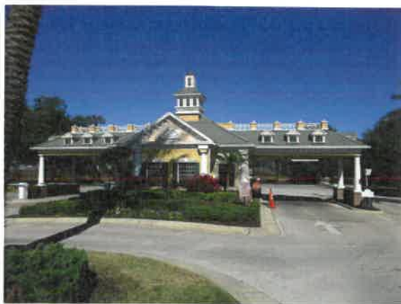
Main gate house
