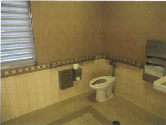
Typical rest room
