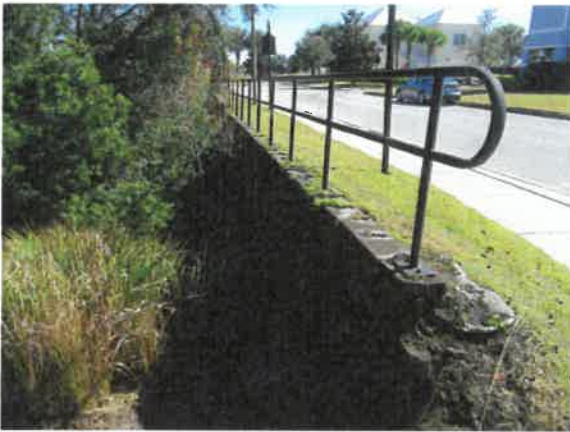
Masonry retaining wall along Reunion Boulevard, note – extensive quantity
