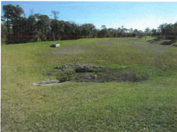
Storm water detention basin at Encore phase
