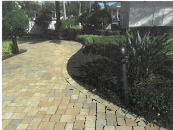
Bollard lights at The Terraces
