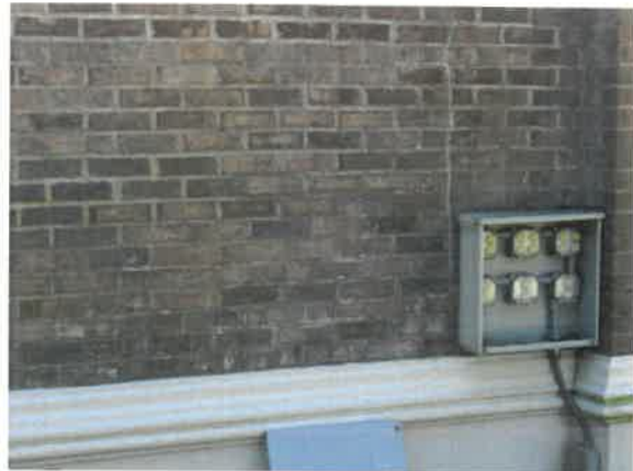
Minor efflorescence
