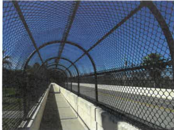
Fencing at Gathering Drive bridge
