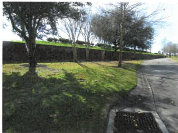
Retaining wall near The Terraces
