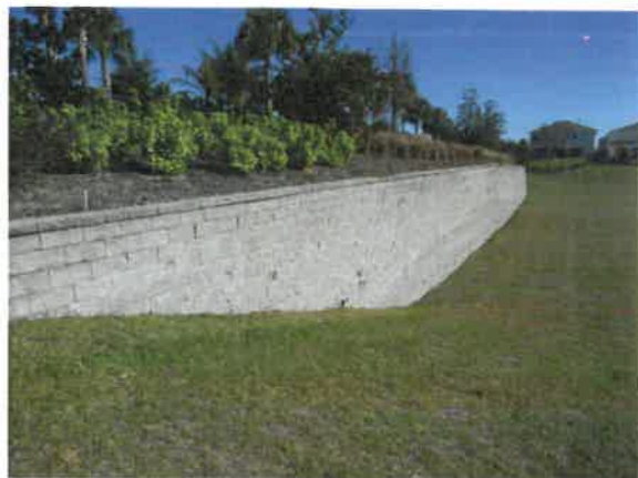
Retaining wall at Encore phase detention basin
